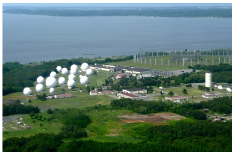
"Hill" complex with Lake Ogawara in background.
